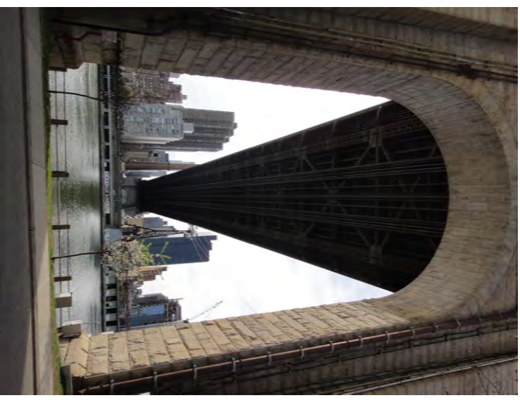
Underneath the Queensboro Bridge
